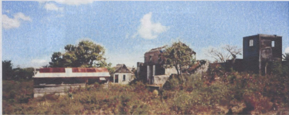
Figure 8.4: Recreation Hall on Left, Office and Staff Quarters on Right; Photo taken in 2000.
