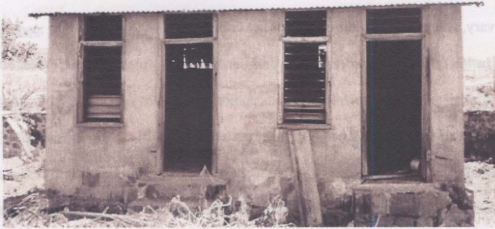
Figure 8.8: Hansen Home Jail; Structure 3; Photo taken in 2000.
